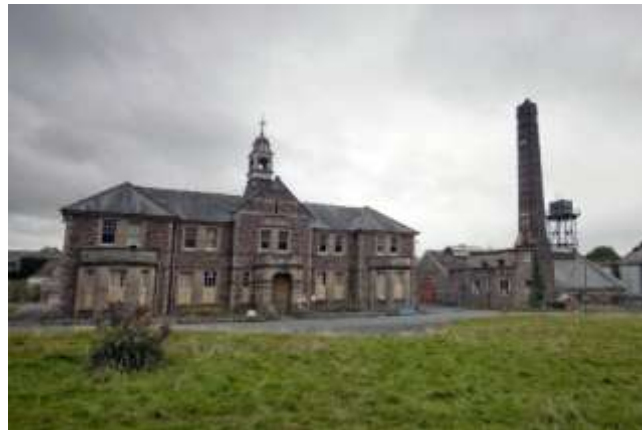
Mid-Wales Hospital, Administrative Block.
