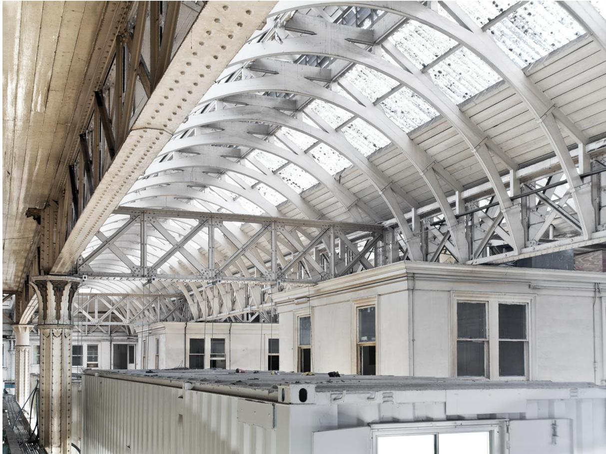
**Photo of Columns, lattice girders and roofing system in General Market. *SAVE Britain's Heritage***
