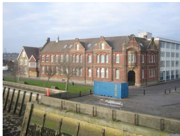
Built in 1903, the A&P building occupies a fine position overlooking the Medway with views towards Rochester Castle
