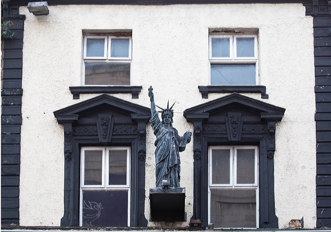
Detail of the former Irish American Bar on Lime Street, set to be demolished as part of the redevelopment proposals.
