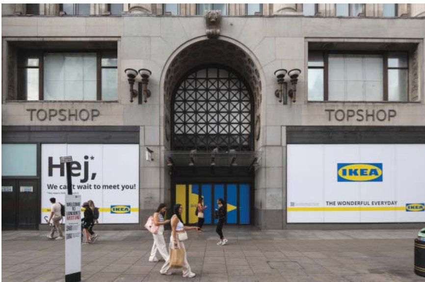
Above: One of the two Beaux Arts style entrances to 214 Oxford Street, formerly the flagship store of fashion brand Topshop. The grade II listed building is soon to reopen as the flagship London store of Swedish furniture giant IKEA. It is one of the many landmark former department stores on Oxford Street being refurbished and converted for new uses (Credit: Stephen Chung /Alamy)
