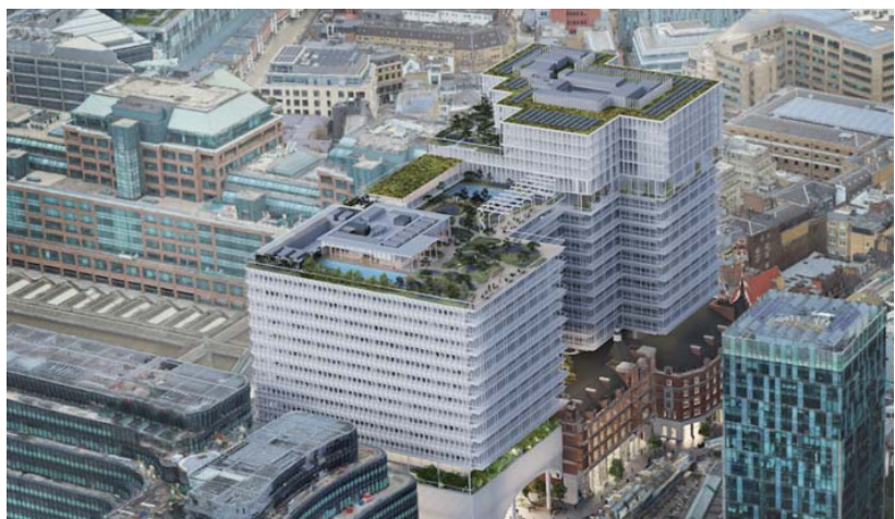
PROPOSED CGI showing an aerial view down onto Liverpool Street with the proposed office and hotel building dumped in place of the existing station concourse and on top of the grade II* listed Great Eastern Hotel (Credit: Herzog & de Meuron)
