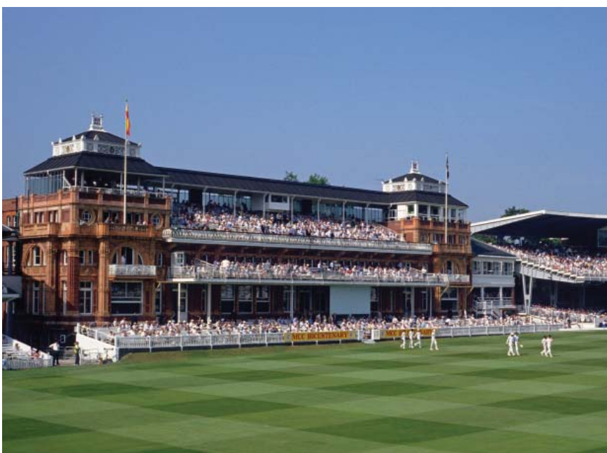
The Pavilion at Lord's cricket ground in north London. Designed by Thomas Verity and completed in 1890, the pavilion is an expression of late Victorian pomp and is now listed grade II* (Credit: Alamy)
