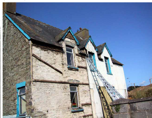
Heolas Fawr on the road to recovery; the above picture shows the removal of corrugated iron cladding
